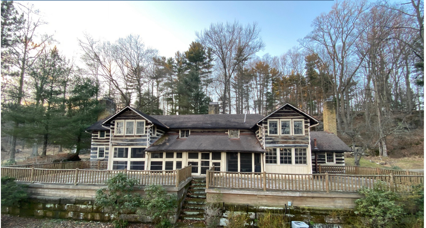
The Heisey cabin as it appears today. Please see the construction-era photo at top of page 9.
