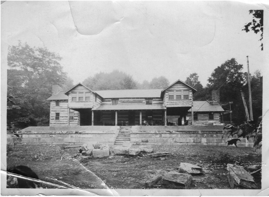
A rare exterior shot of the cabin during construction
