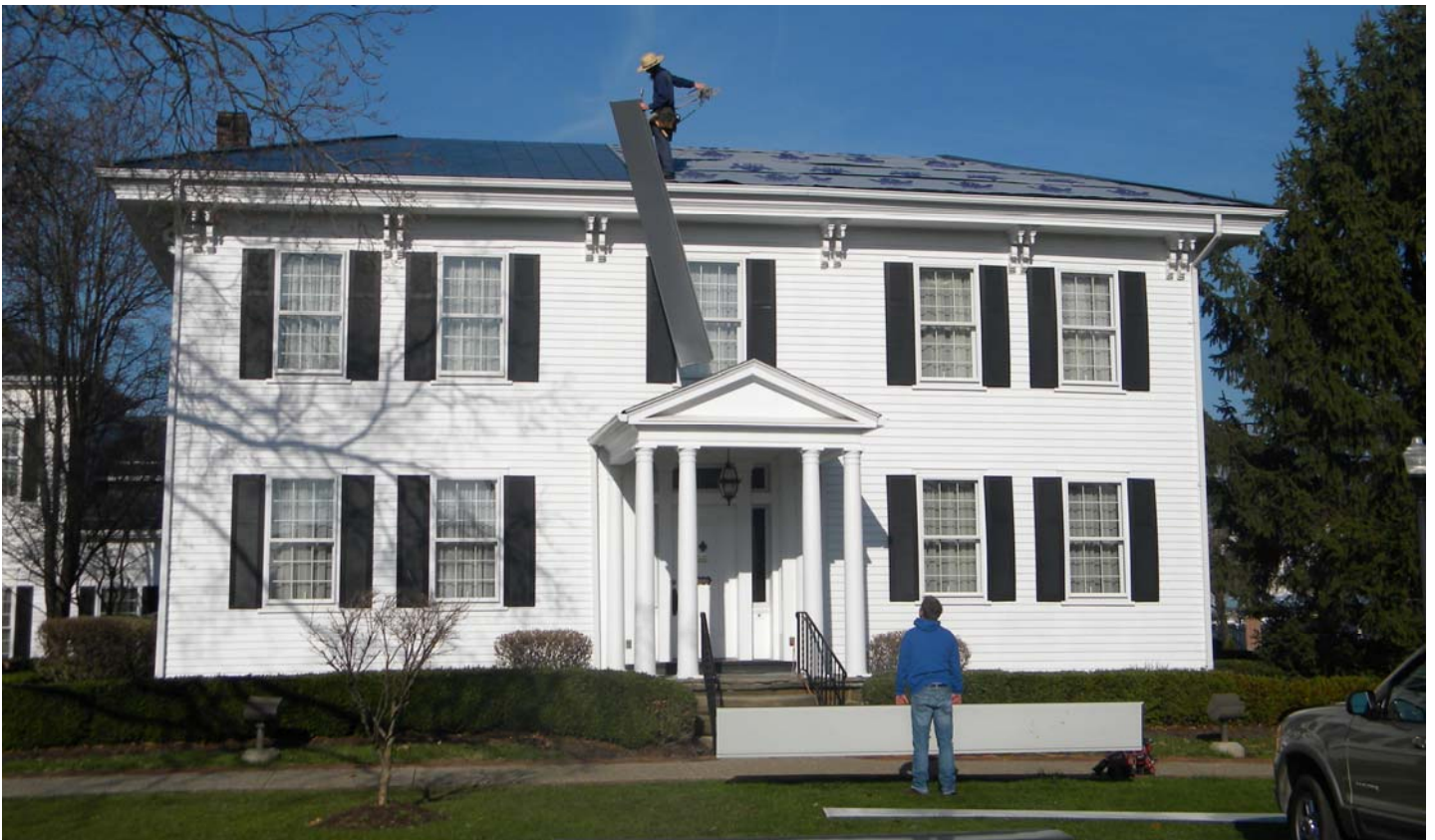
King House Receiving Its New Roof
