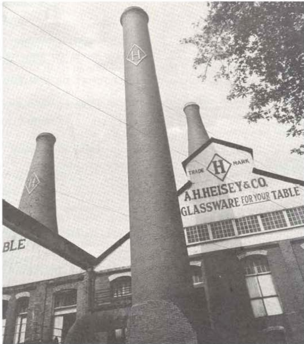
Factory Smokestacks before They Were Taken Down (See Story Page 20)
