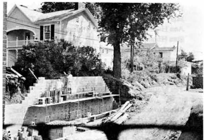
Each day the cement block walls grew. Photo by S. Pennington
