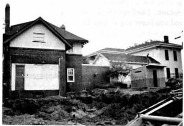
North view of backyard--Porch is gone. Photo by S. Pennington
