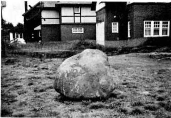
Buried treasure! This rose granite boulder was unearthed during excavation. It will be saved and will be incorporated into the new courtyard landscape design. Photo by S. Pennington
