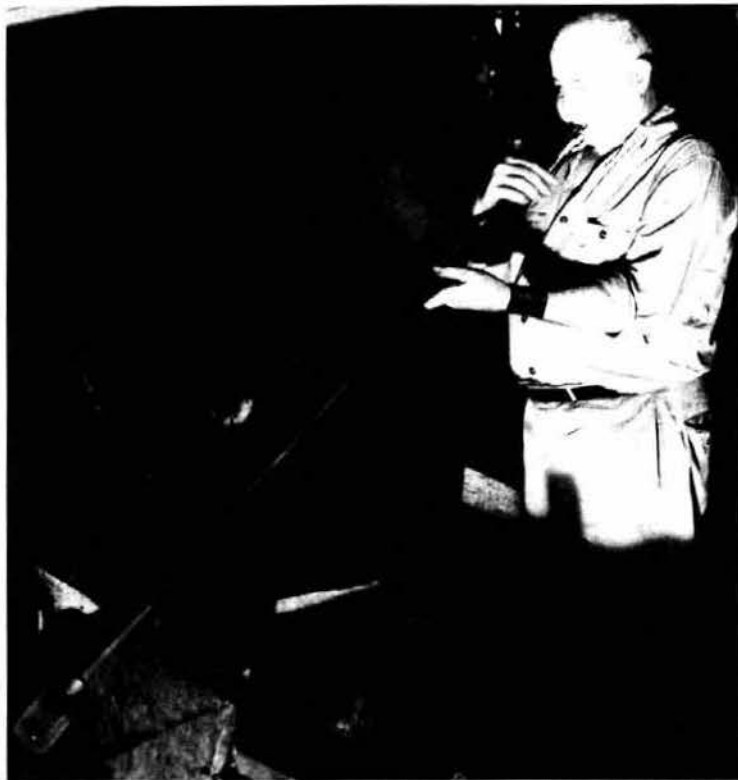
THE BLOWER BEGINNING TO BLOW GLASS THROUGH THE HOLLOW BLOWPIPE.
