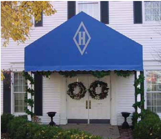
The New Awning
