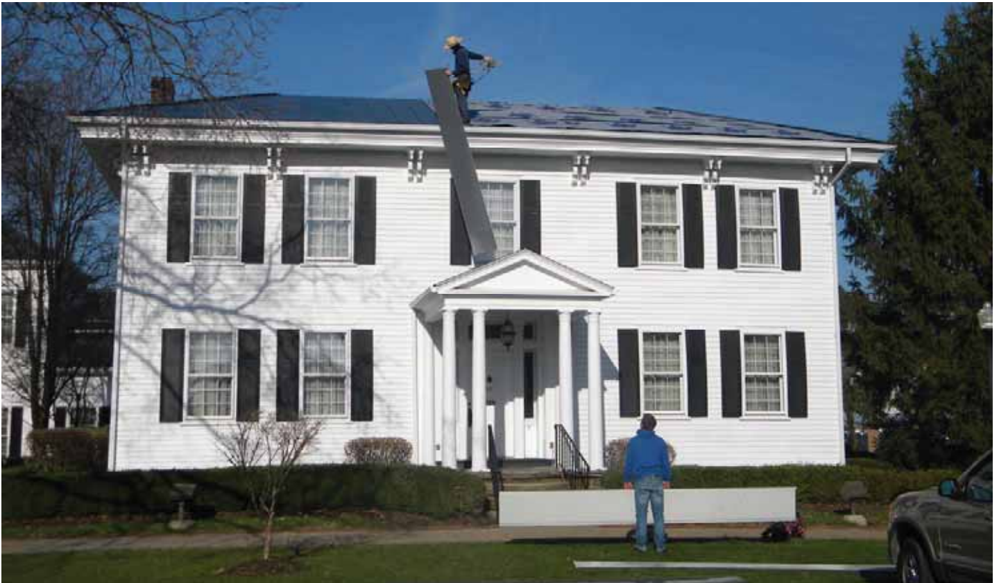
King House Receiving Its New Roof
